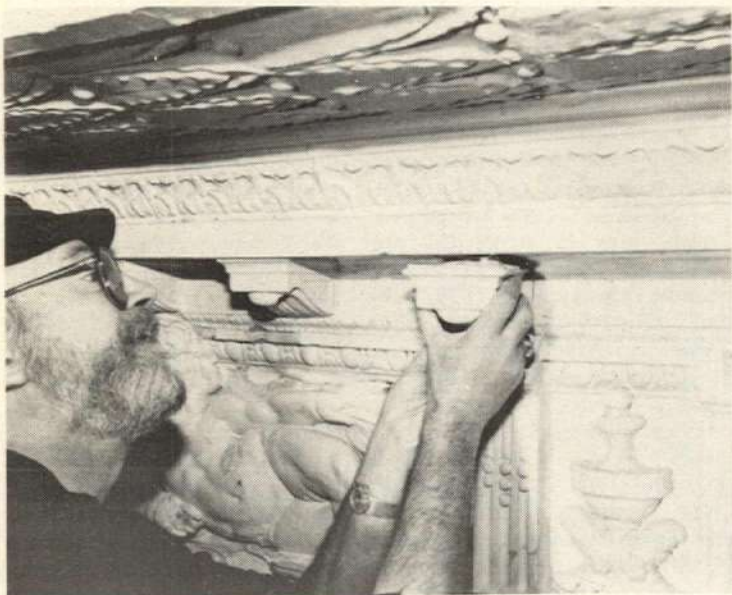
Restoration of the ceiling mouldings in the lobby of the Elgin Theatre, February 1985. Photo courtesy Gary Beechey, Elgin/Winter Garden Unit, Ministry of Culture & Communications.
