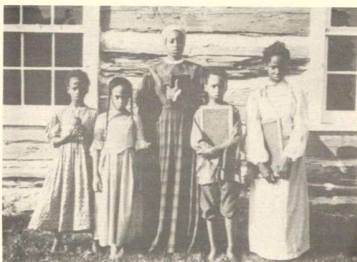
Photo used in production of the Ontario Black History Society's video. (See article below for further details.) Photo courtesy National Film Board.
