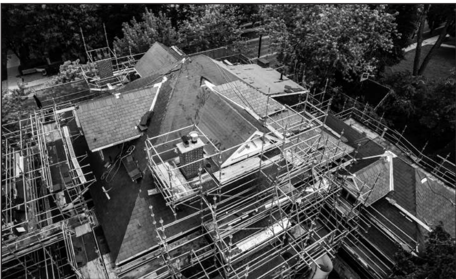
Slate roof restoration at John McKenzie House in 2016.
