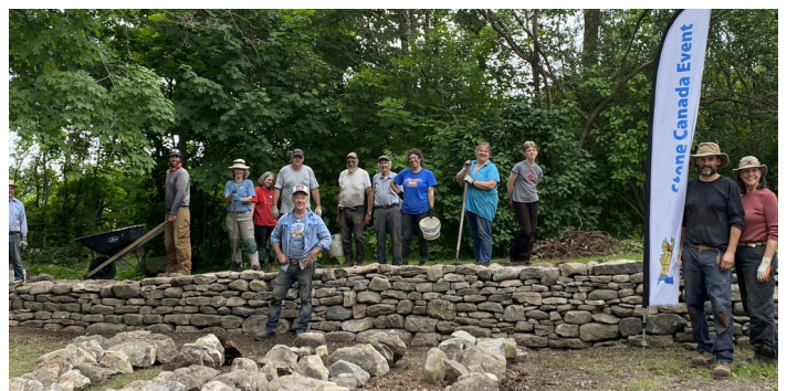
Volunteers assembled in 2020 to help restore the stone wall.
